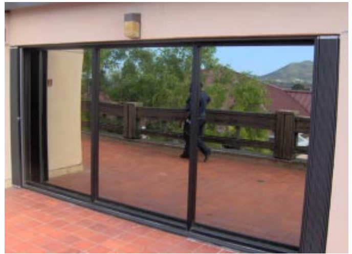
Arthur Joseph, supervisor of maintenance at UVI, is reflected in the new windows.
